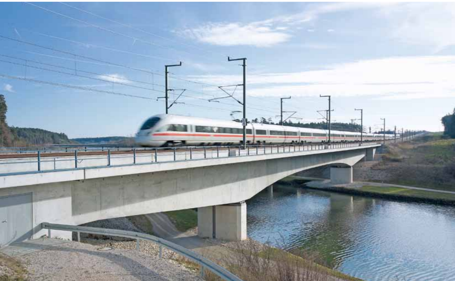
Newly built railway line Nuremberg – Ingolstadt – Viaduct Main – Danube – Canal
